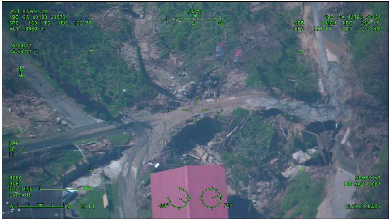
Figure 13 Damaged Road in Puerto Rico
