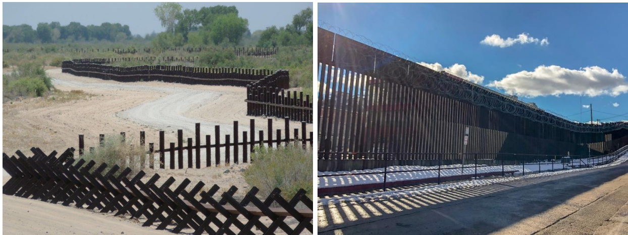
Figure 2. Left , example of a vehicle barrier; right , example of a pedestrian barrier
