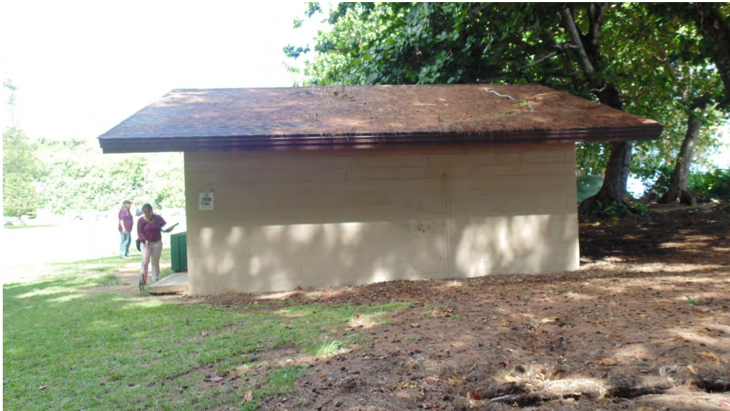
Figure 11 DOPR intern with measuring wheel at a comfort station in Anini Beach Park
