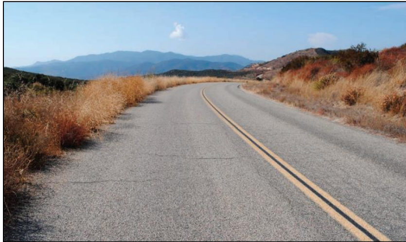
Figure 14. Maintenance Level 5 USFS Road
