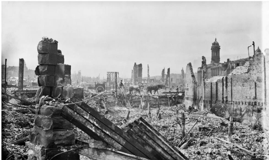
Figure 3. Total devastation in the 1906 San Francisco ~7.9 earthquake
