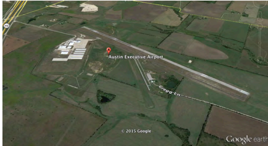
Figure 11 Aerial imagery of study area from Google Earth
