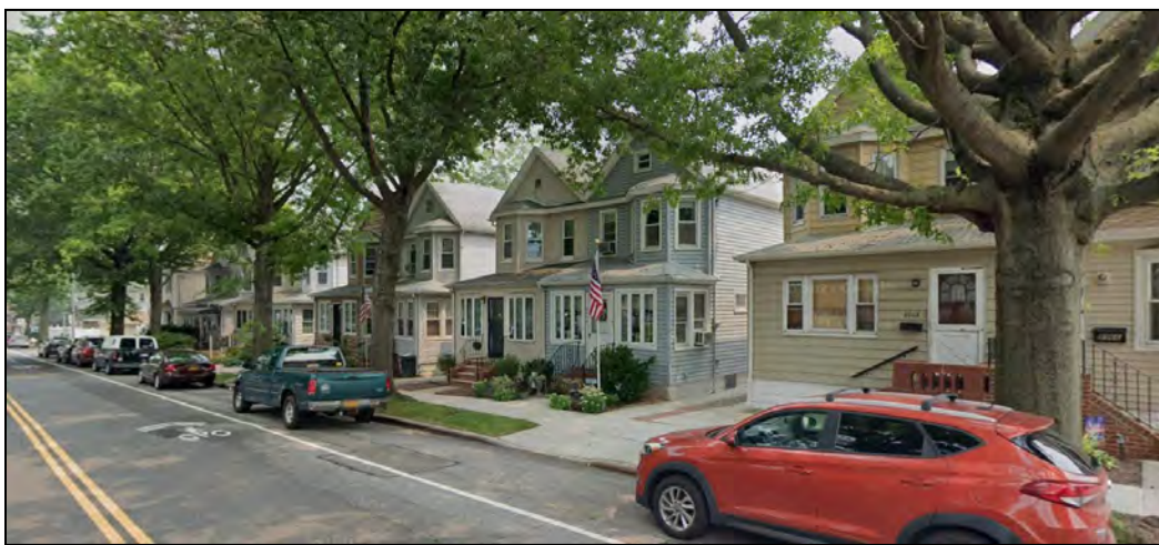
Figure 37. Semi-detached homes in Queens (Google 2022)
