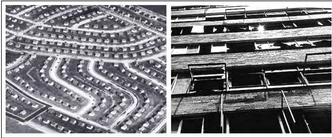
Figure 12. Different trajectories stemming from the Housing Act of 1949 (Levittown, NY, 1950s, and Pruitt-Igoe, St. Louis, 1960s) (Sheidlower 2020; Newman 1996)
