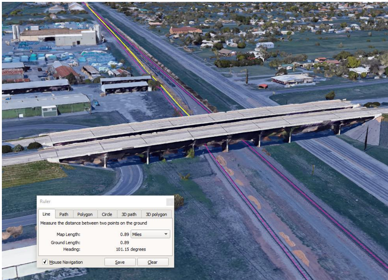
Figure 23 – Google Earth Railroad Use Case Bridge Violation
