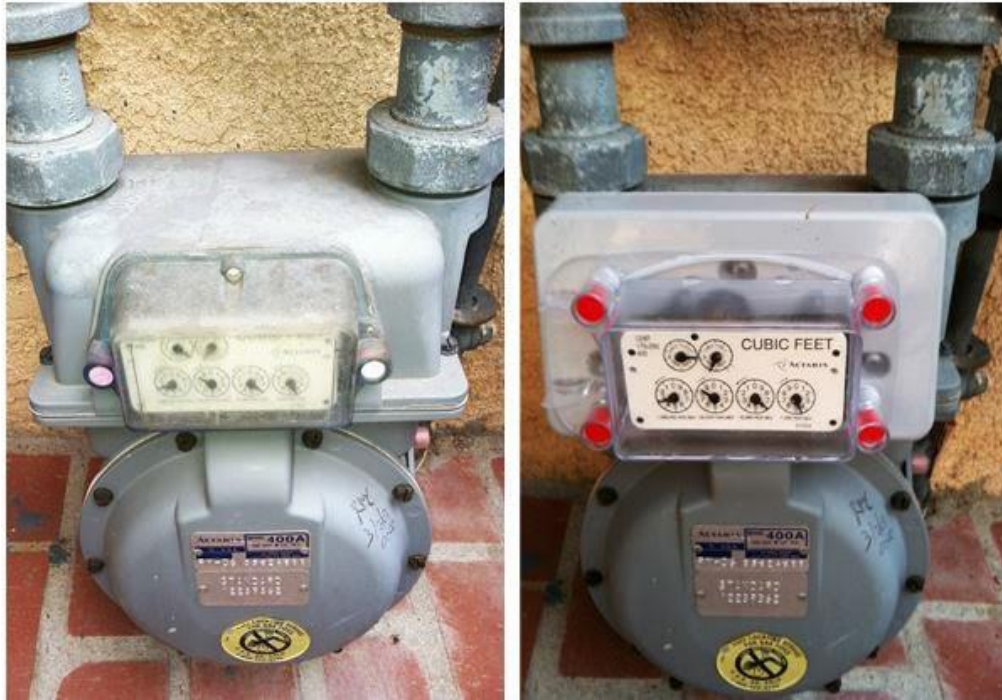
Figure 2: Standard gas meter (left) and smart grid utility meter (right)
