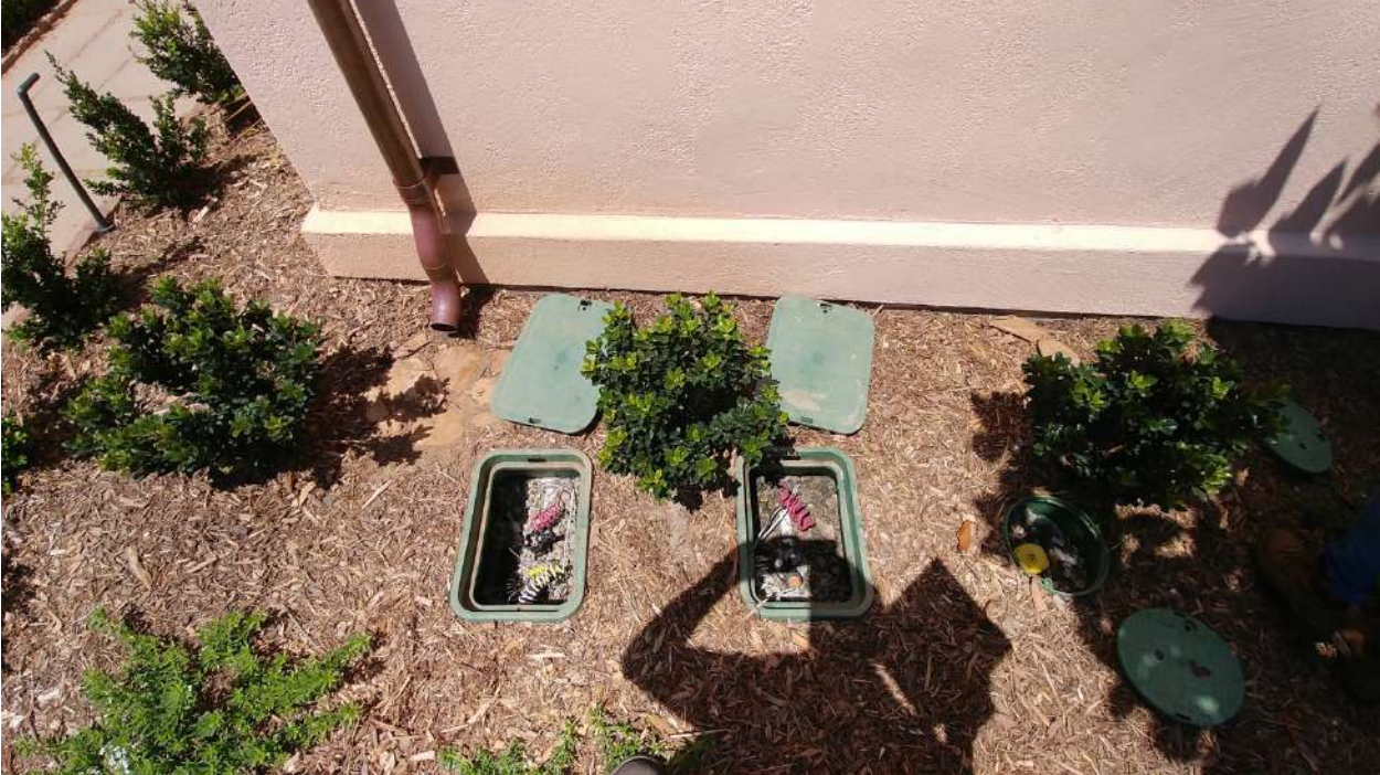
Figure 3: Field photo of two remote control valves (left) and a quick coupling valve (right)
