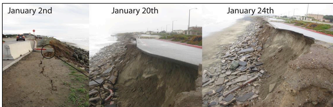
Figure 4 - Coastal erosion from January 2-24, 2010 from storm surges in San Francisco ( https://www.usgs.gov/media/images/coastal-erosion-san-francisco-0 )
