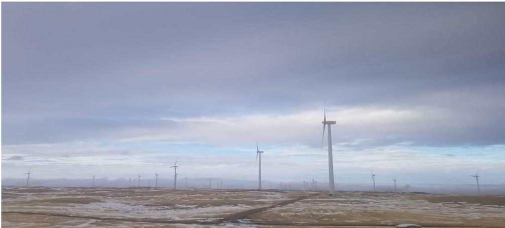
Figure 3 - Turbine array with tubular style turbines. Photo credit: Andrew Burmester.
