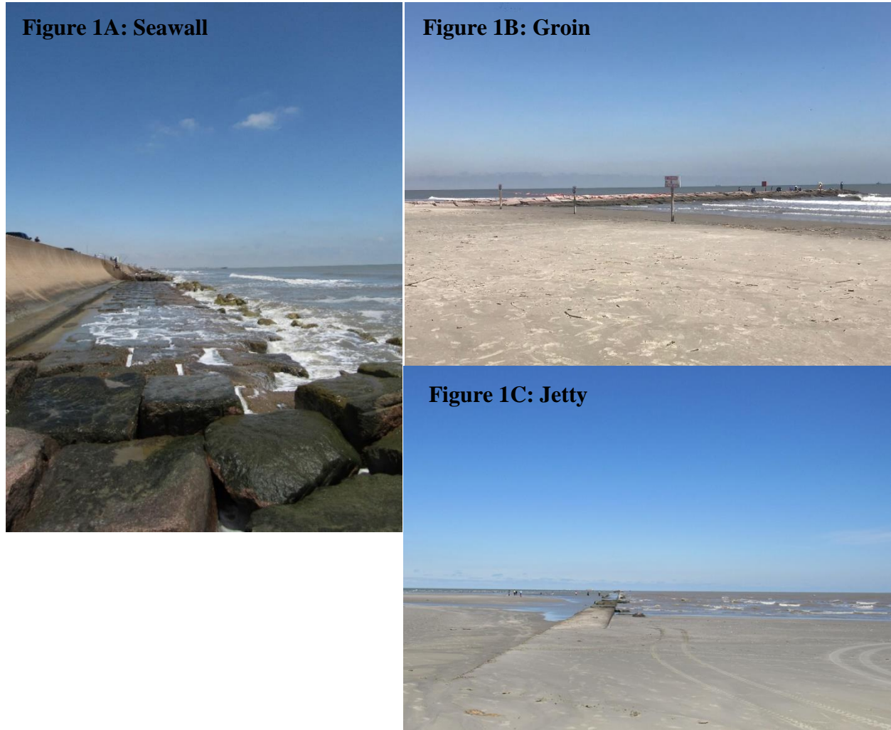
Figure 1: Photographs of the coastal structures defining Galveston's coastline taken by Michael Thibodaux
