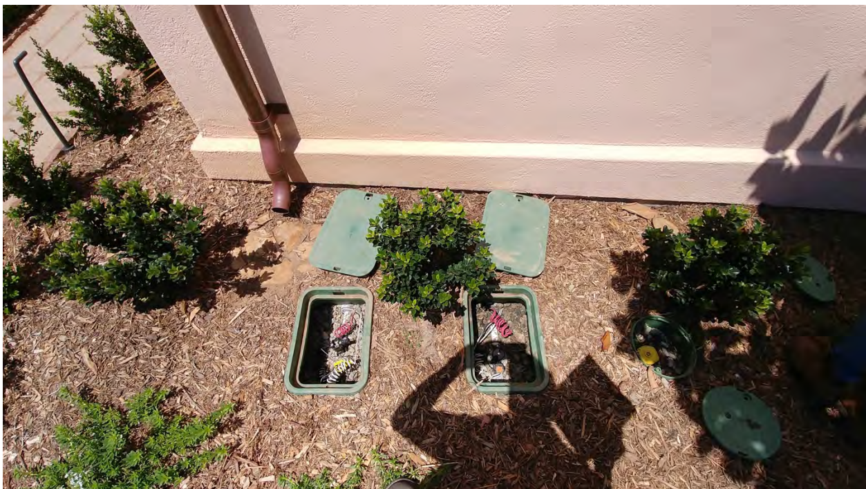
Figure 3: Field photo of two remote control valves (left) and a quick coupling valve (right)
