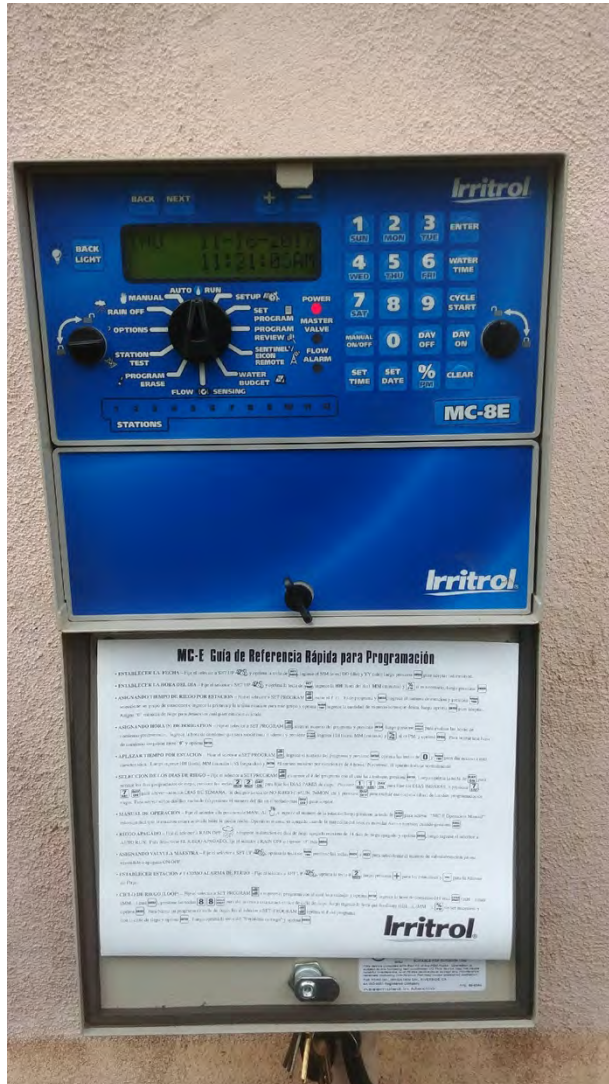
Figure 4: Field photo of controller D, a wall-mounted Irritrol box with up to 12 connections
