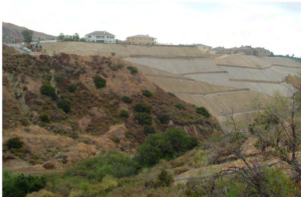
Figure 7. Hillside modifications along Aliso Canyon Wash Park
