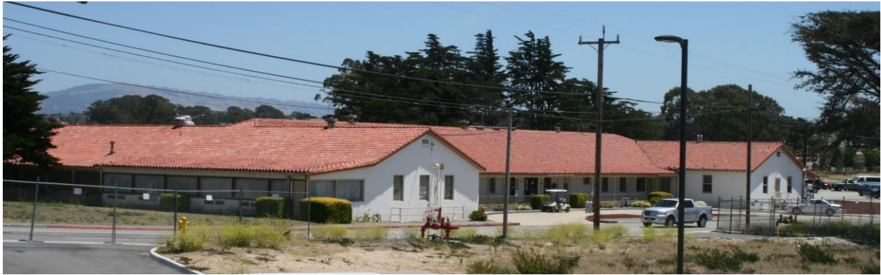
Figure 16 Building 2798, Martinez Hall
