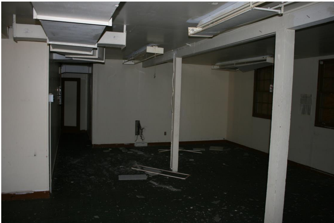
Figure 24 Building T-2906 interior 1
