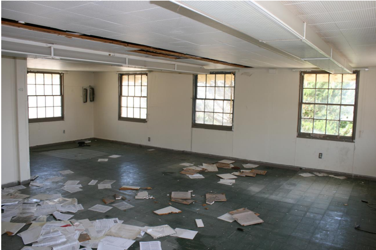
Figure 25 Building T-2906 interior 2
