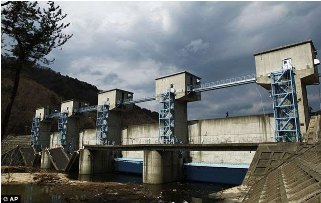
Figure 34. Fudai Seawall (Adapted from the Associated Press 2011)
