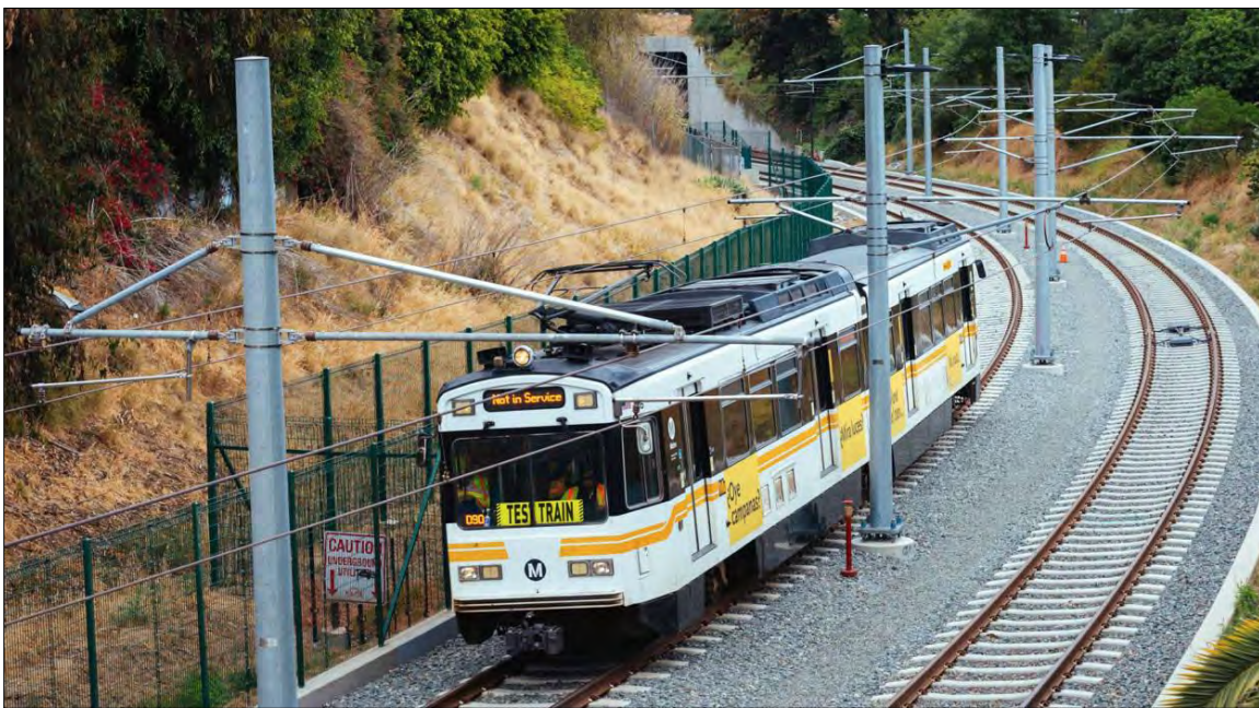
Figure 12 OCS supplying electricity to the LR train. Source: Metro Source 2015
