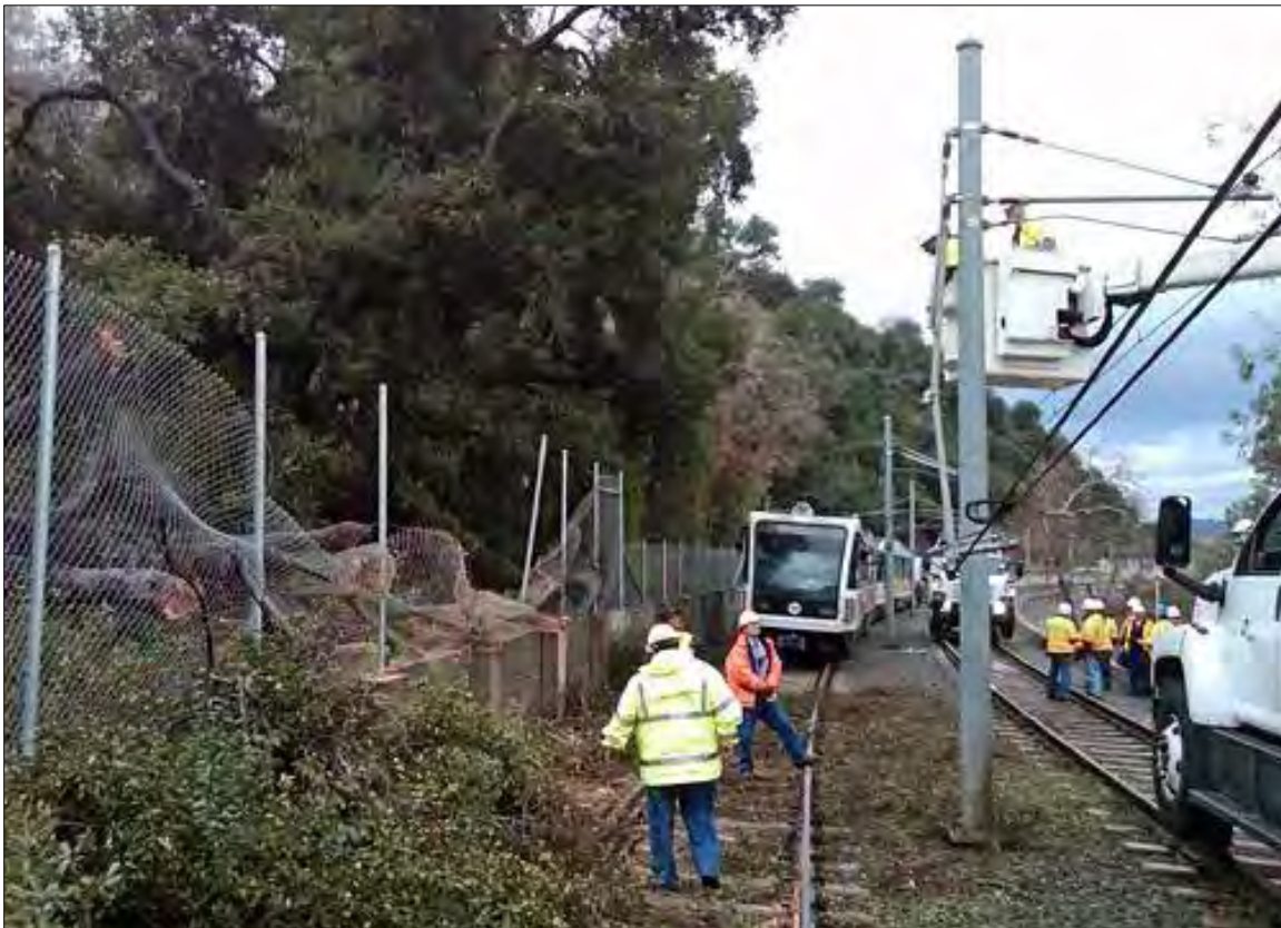
Figure 10 Traction Power personnel repairing Gold Line OCS cables with the aid of Hi-Rail vehicles. Source: Metro Source 2010
