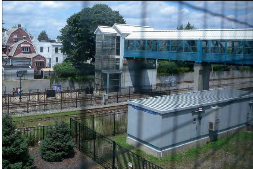
Figure 11 TPSS building (lower right) near the train tracks. Source: Wikimedia Commons 2015
