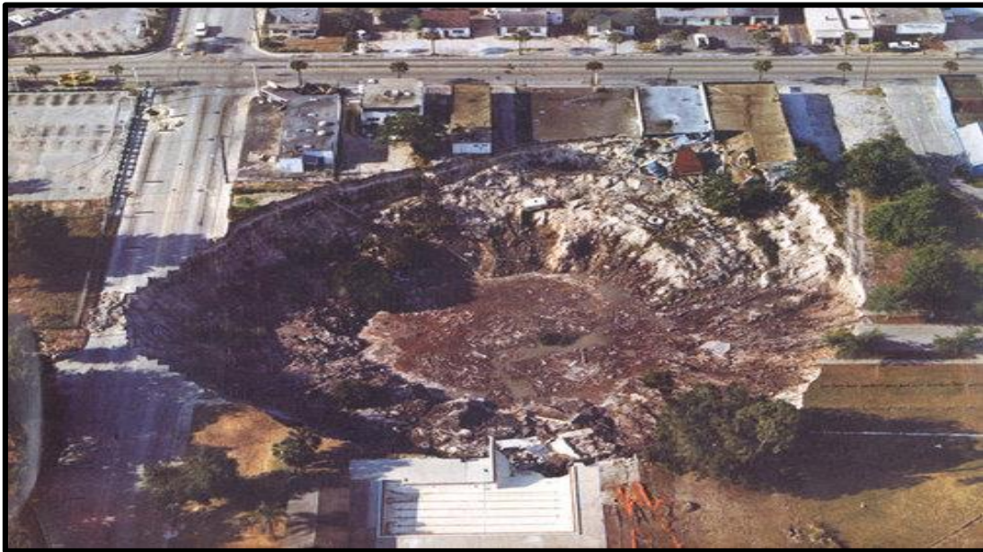
Figure 4 Aerial view of the Winter Park Sinkhole (Orlando Sentinel 1981)
