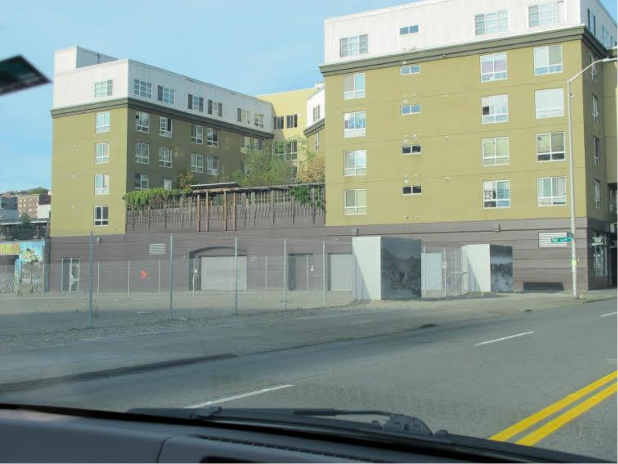
Figure 32 Ground view of 1250 Denny Way
