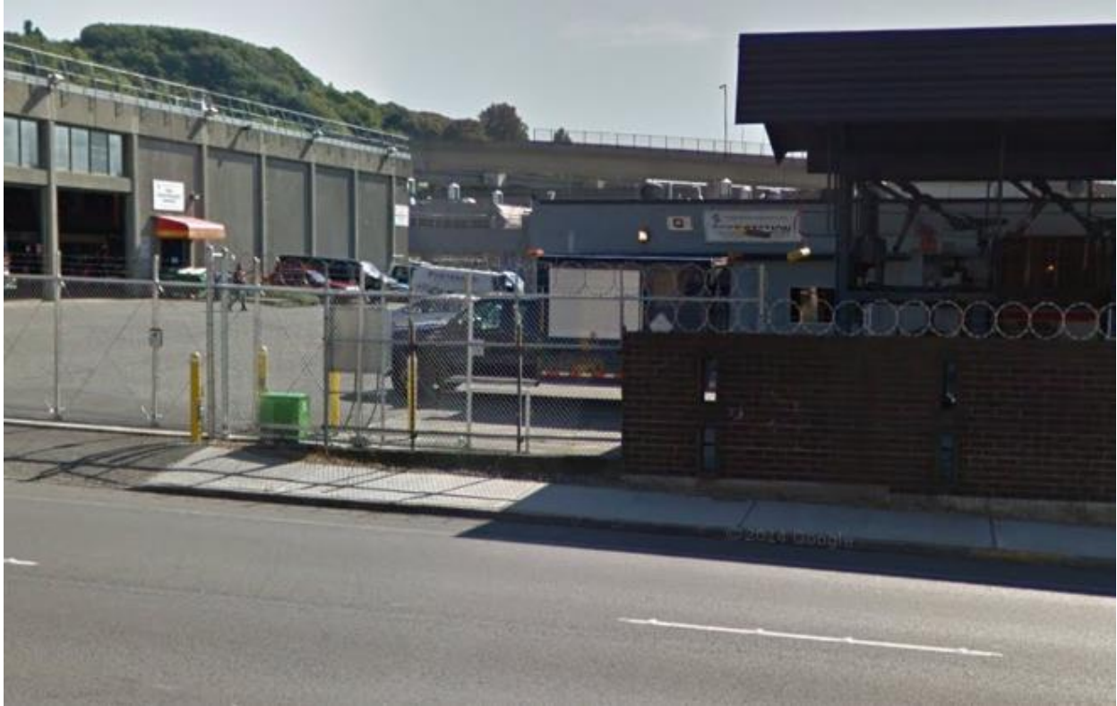
Figure 26 Ground view of 801 South Dearborn Street
