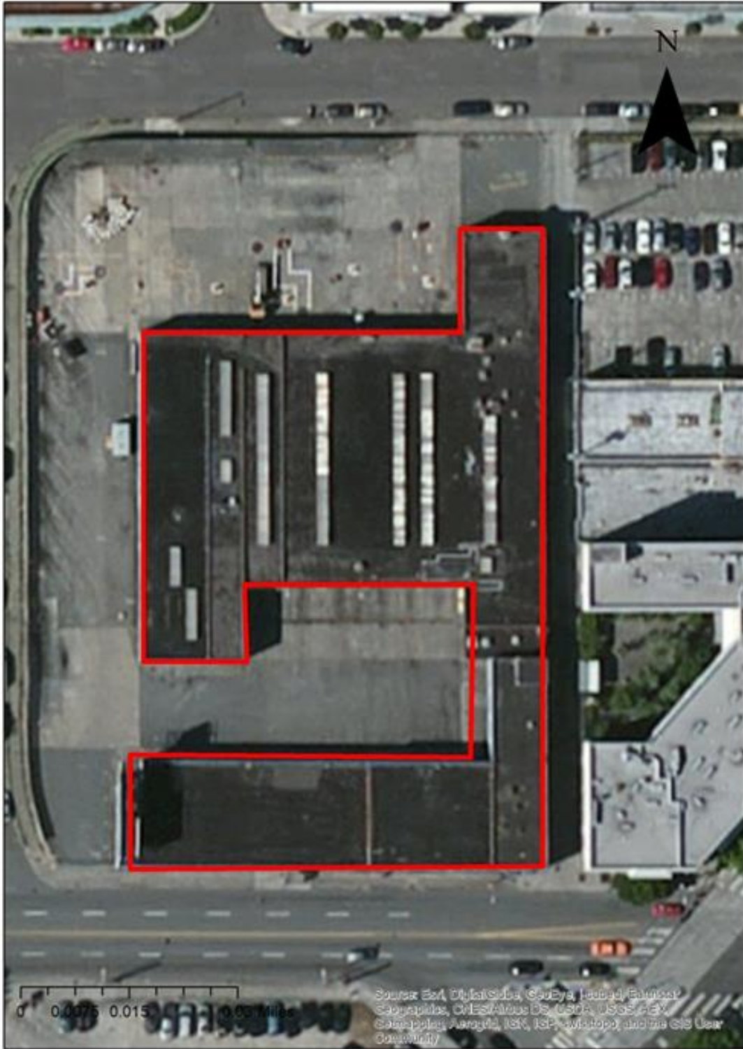
Figure 31 Aerial view of 1250 Denny Way
