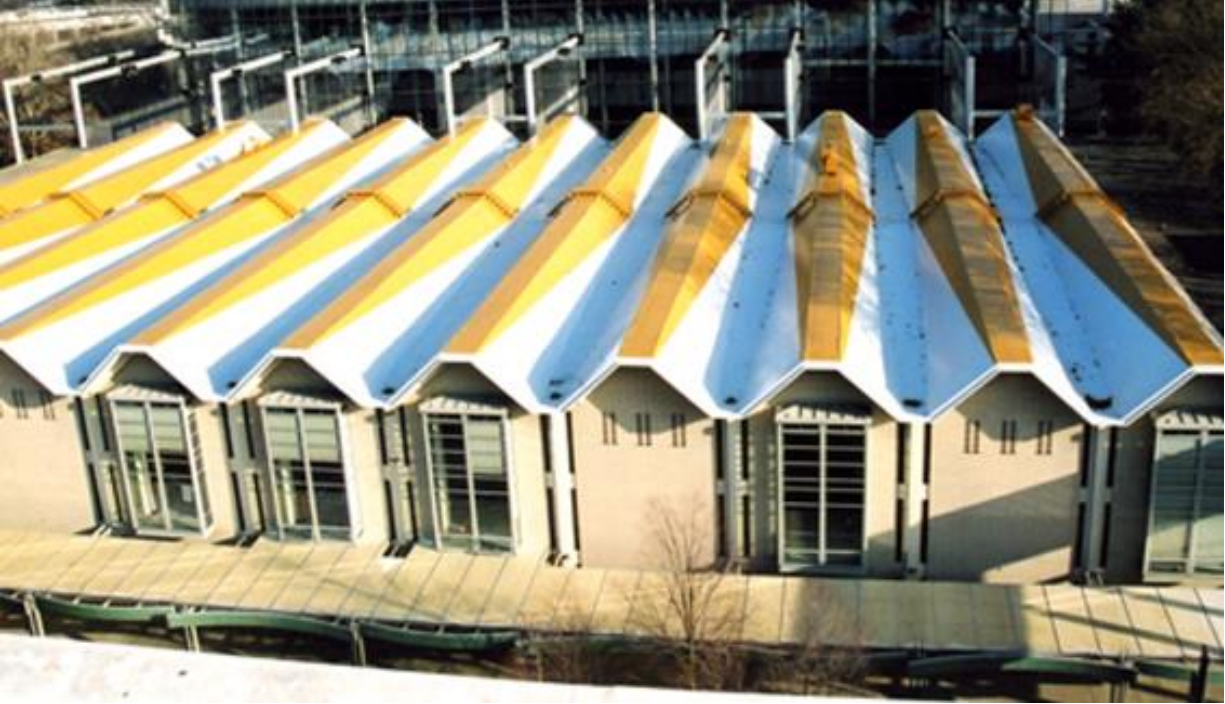
Figure 24 Aerial view of 301 Mercer Street displaying the roof's rolling geometry Photography by Public47 Architects
