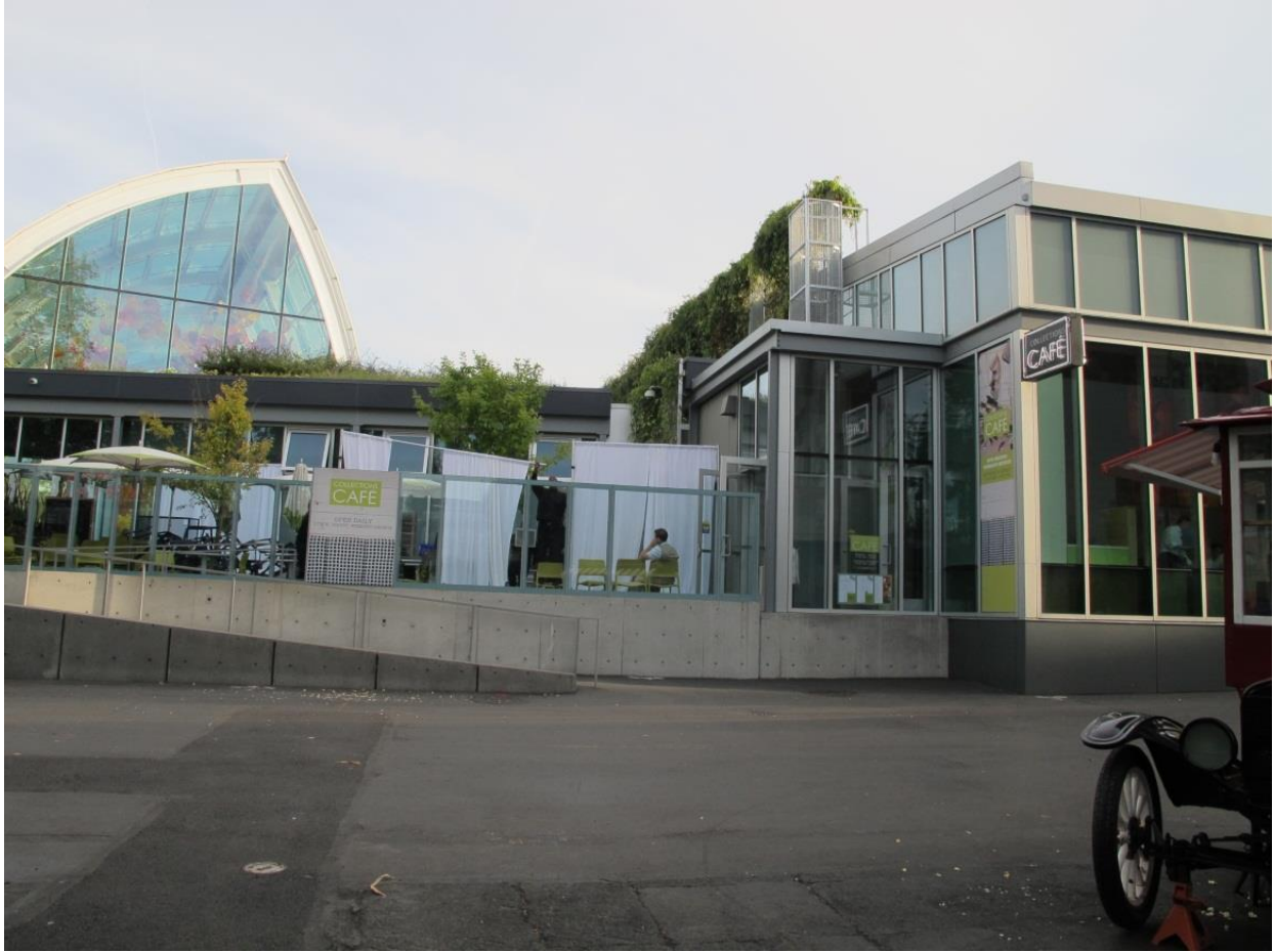
Figure 20 Ground view of 305 Harrison Street
