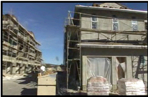
(c) Under Construction
