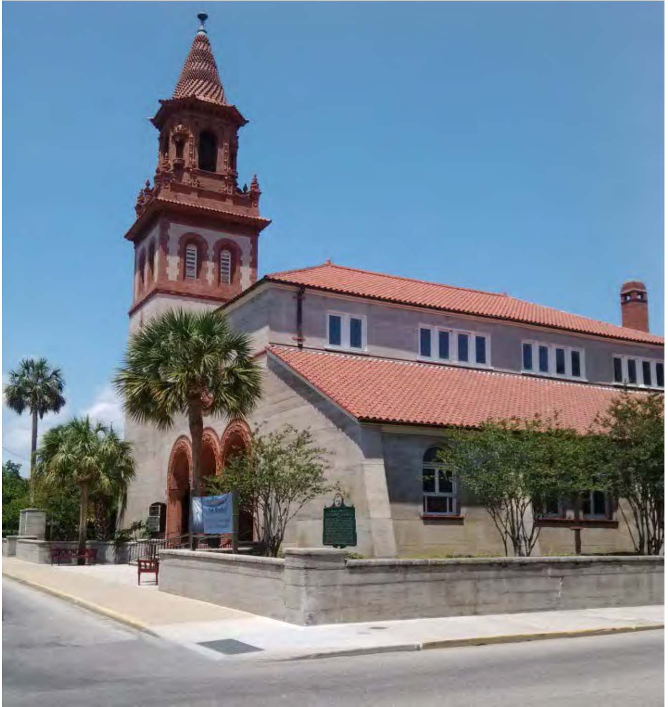
Figure 5: Grace United Methodist Church. Built by Henry Flagler in 1886 to replace the original structure occupying the desired site of the Hotel Alcazar, it was the second structure in St. Augustine to be built using the Poured Concrete method (note the horizontal striations in the walls caused by the molds used when pouring and setting the concrete)
