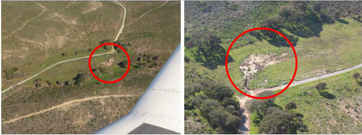
Figure 25: Erosion Scars Assisted in the Confirmation of Site ID# 80P07 as a CVP (Photo Credits: C. Hanley)
